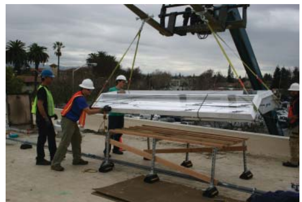
SunWater Solar installers bring MCT collectors to the roof
